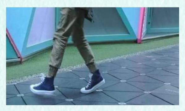
Pavegen is a company that specializes in creating innovative flooring technology. They develop a type of flooring that generates electricity from human footfall. As people walk over the Pavegen tiles, the pressure from their steps causes the tiles to flex, generating small amounts of kinetic energy that can be converted into electrical energy. This concept is often used in high-footfall areas like urban spaces, shopping centers, and transportation hubs to harness energy from pedestrian movement.
